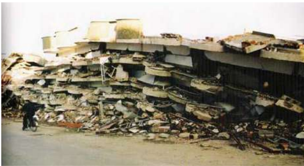
Figure 14. Damage due to the hollow-tile floor slab [Photo by Elif Çiftçi]
