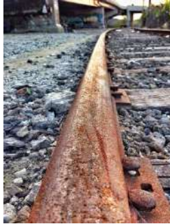
Figure 7. An example of oxidation defect that can happen in the rail [19].
