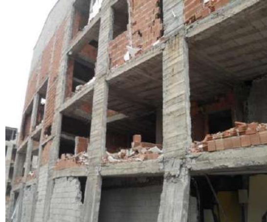
Fig 2. A damaged building with hollow block slab after Van earthquake (2011)
