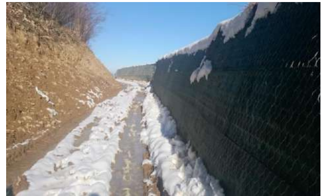
Fig. 5. Compacted soil and reinforced embankment wall at Araklı Yeşilyurt
