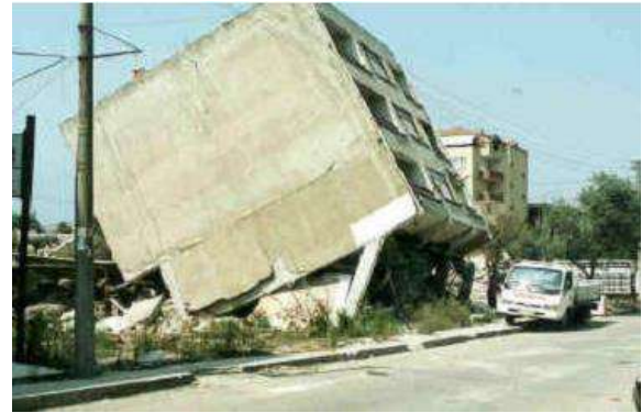
Figure 8. Damage due to the heavy cantilevers [Photo by Kutlu Darılmaz]
