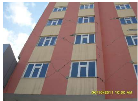
Figure 13. X cracking due to the short column
