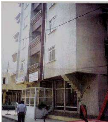
Figure 11. Gusseted column damage [Photo by Elif Çiftçi]
